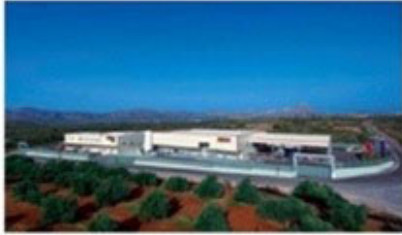
Central facilities – Factory in Chania – Crete- Greece
