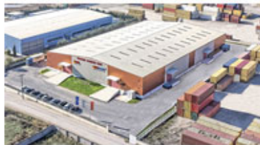
Warehouse in Thessaloniki - Greece
