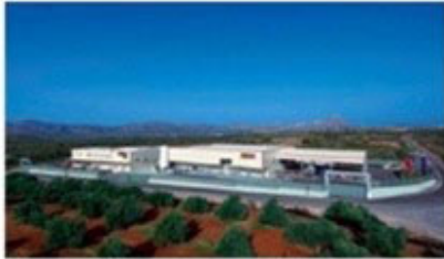
Central facilities – Factory in Chania – Crete- Greece
